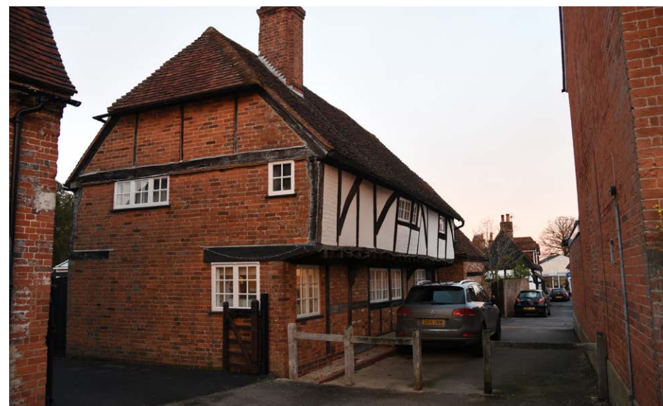
View of Stoney Cottage from the Bury
