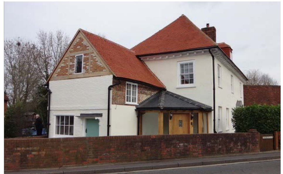
Timber framing on the side elevation and stucco on the front elevation of Nevills, Hook Road
