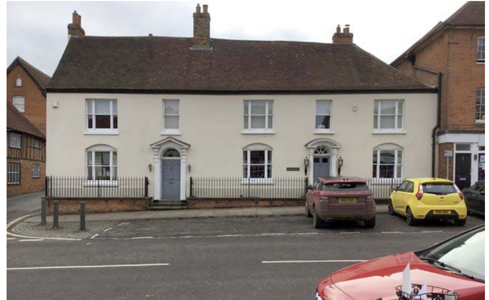
Nos. 67-69 High Street. The re-fronted north façade of a major 15th-century courtyard house
