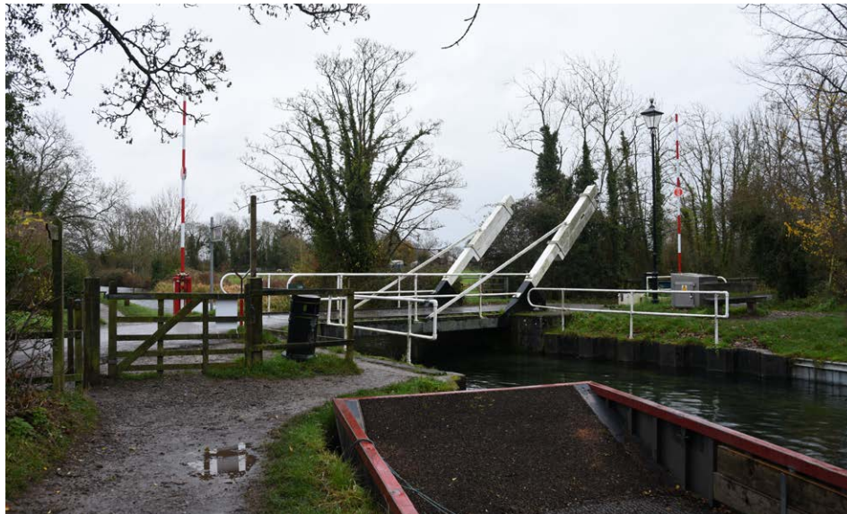
Swing Bridge over the canal
