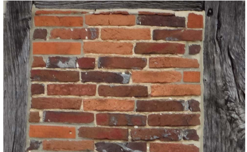
Brick nogging between timber framing on Castlebridge Cottages
